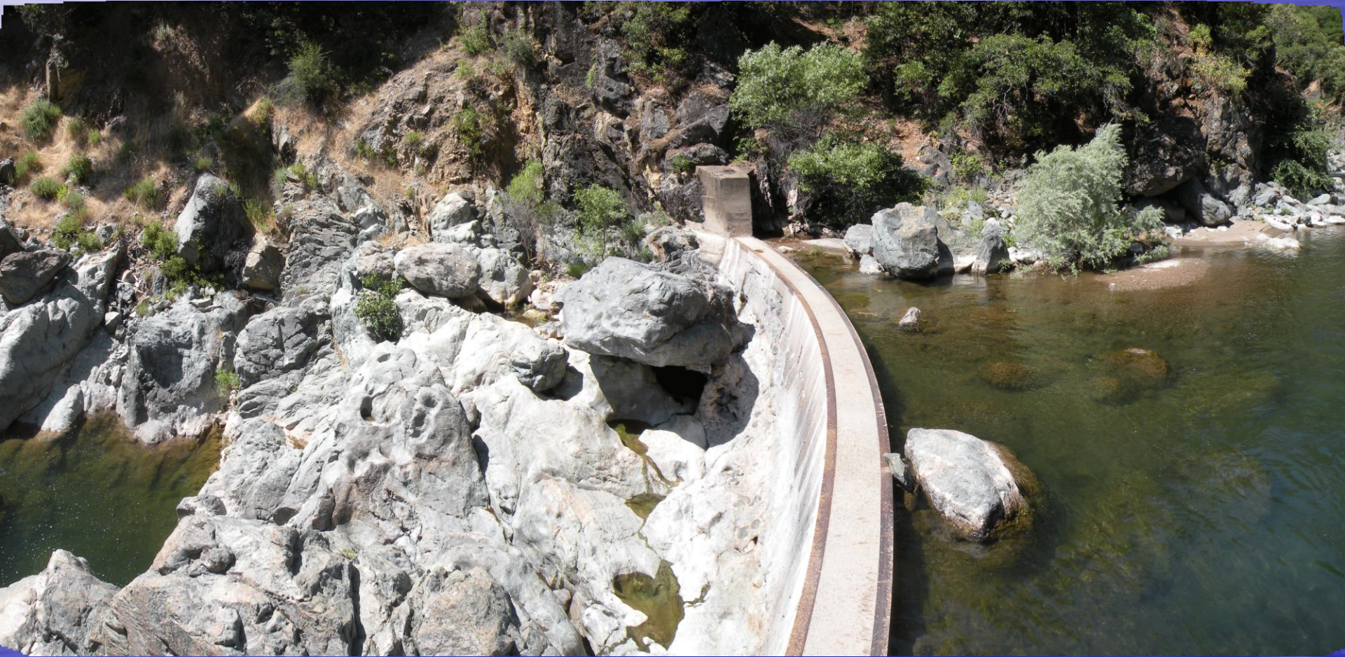
Centerville Head Dam 1150 feet elevation
