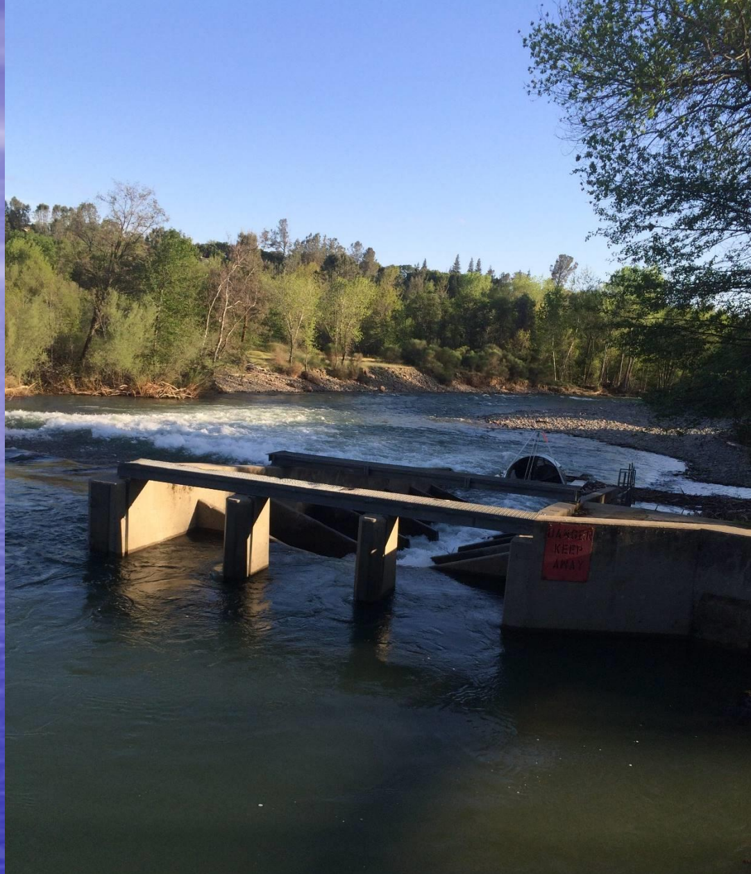
Fish ladder/irrigation diversion
